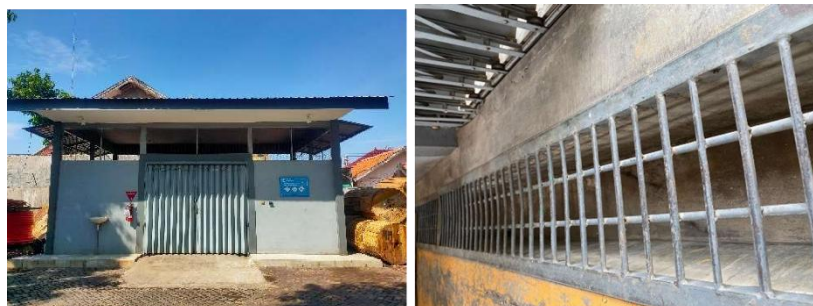
Figure 8 Hazardous Waste Storage at UP3 Pasuruan, 2024
