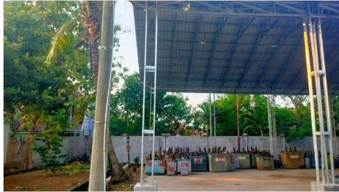
Figure 7 UID Jatim Transformer Warehouse Condition, 2024
