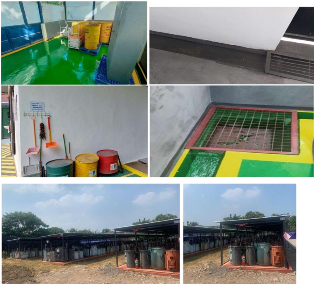
Appendix 11 : No Oil Seepage from Transformation and Empty Transformation Photos
