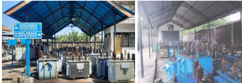
Figure 5. Transformer Warehouse Existing Condition, 2024
