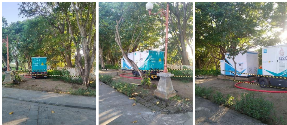
Figure 4. Police Line as a Work Sign, 2024
