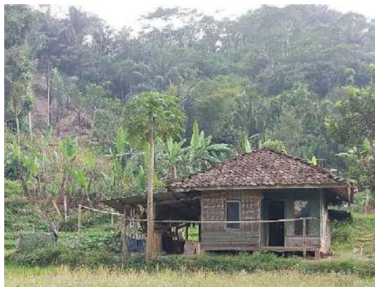
Picture C.1 Residential buildings affected
