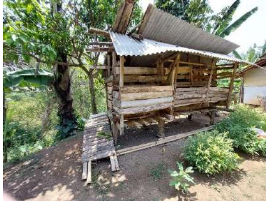
Picture C.2 Stable building affected
