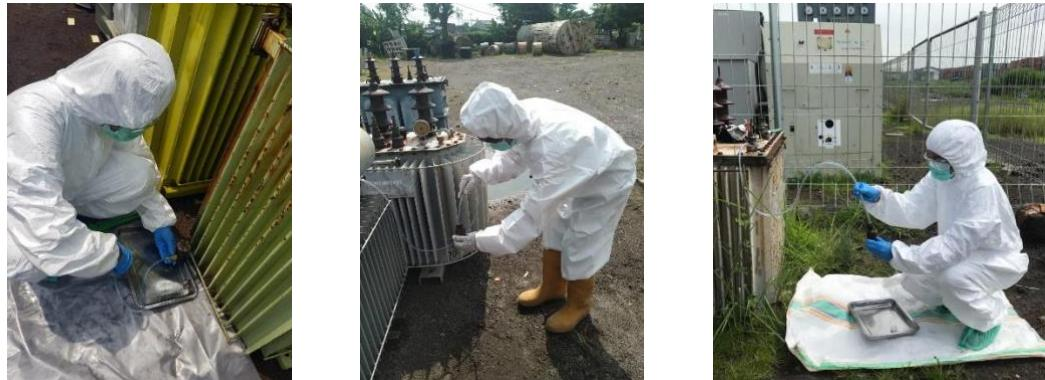
Figure 6. Transformer Offline Oil Sampling for PCBs Test
