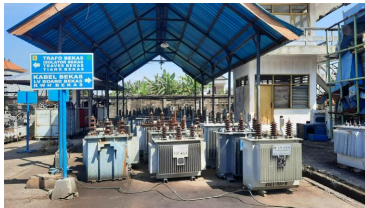
Figure 5. Transformer Warehouse Existing Condition
