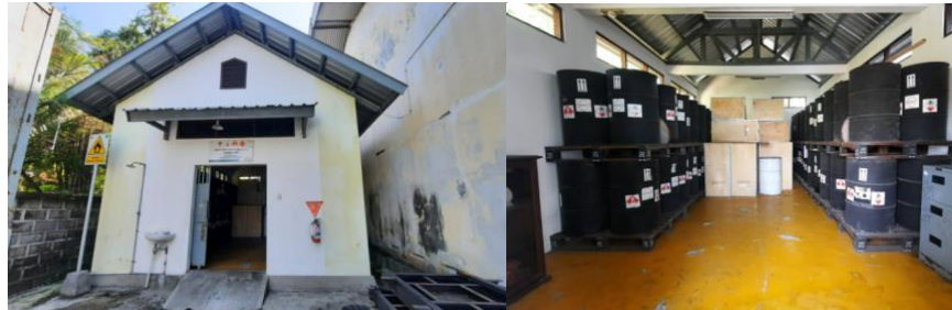
Figure 6. Hazardous Waste Temporary Storage
