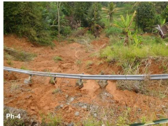
Landslide material is composed of reddish silt and clay
