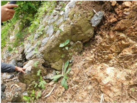
Void behind retaining wall
