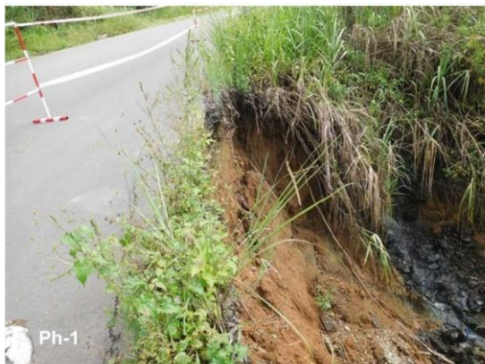
Top of collapse, no more significant cracks
