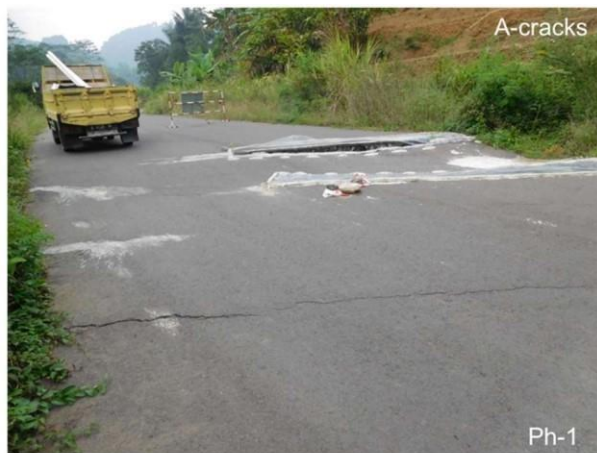
A-cracks featured on road
