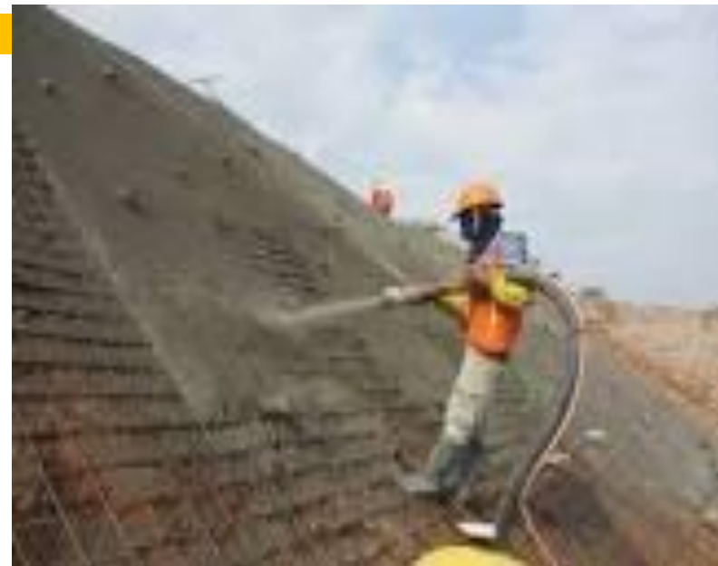
Shortcrete was chosen because it was an emergency job and had to be finished quickly
