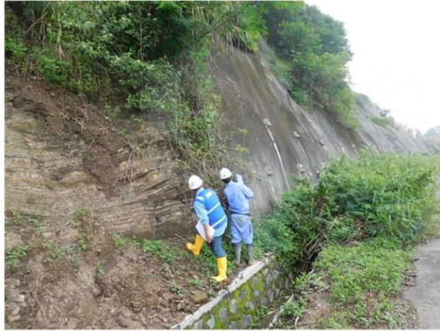
Shotcrete and rock bolt suddenly quit at slid slope
