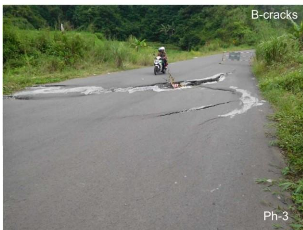
B-cracks featured on road
