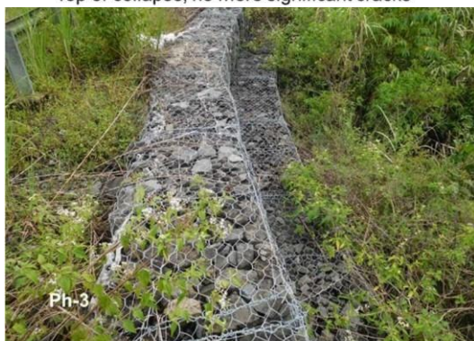
Gabion next to collapse slope
