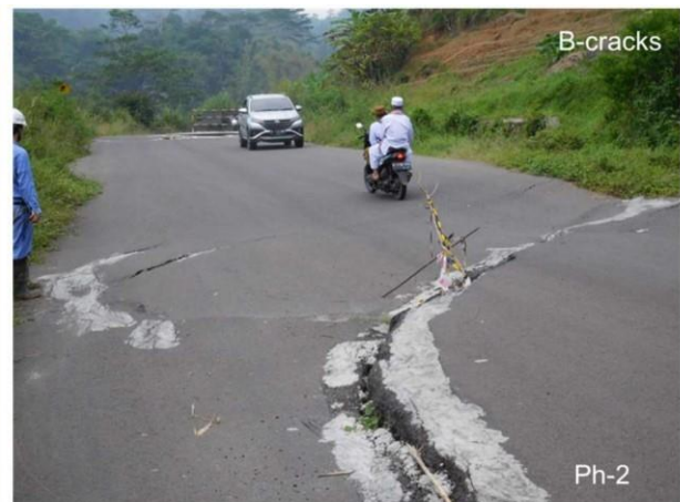
B-cracks featured on road
