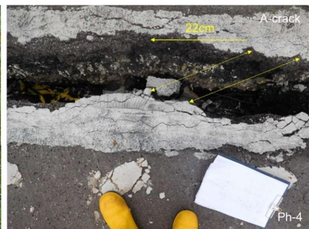
Horizontal displacement: 22cm? Vertical displacement: 14cm
