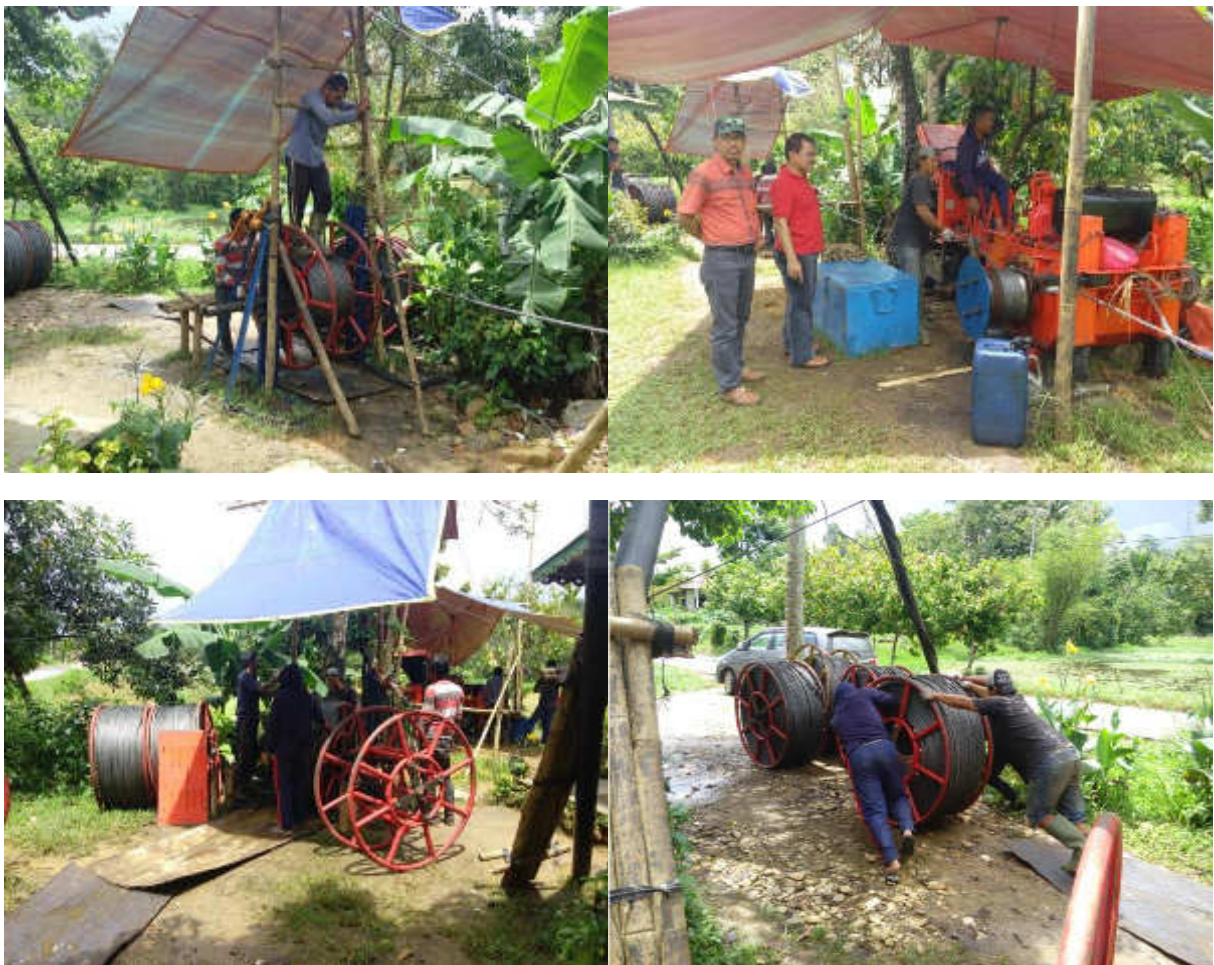
Figure 10 : Whitdrawal Cable Condition
