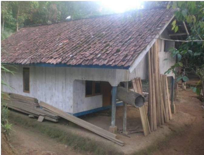
The entire mosque building is made of wooden with roof tiles
