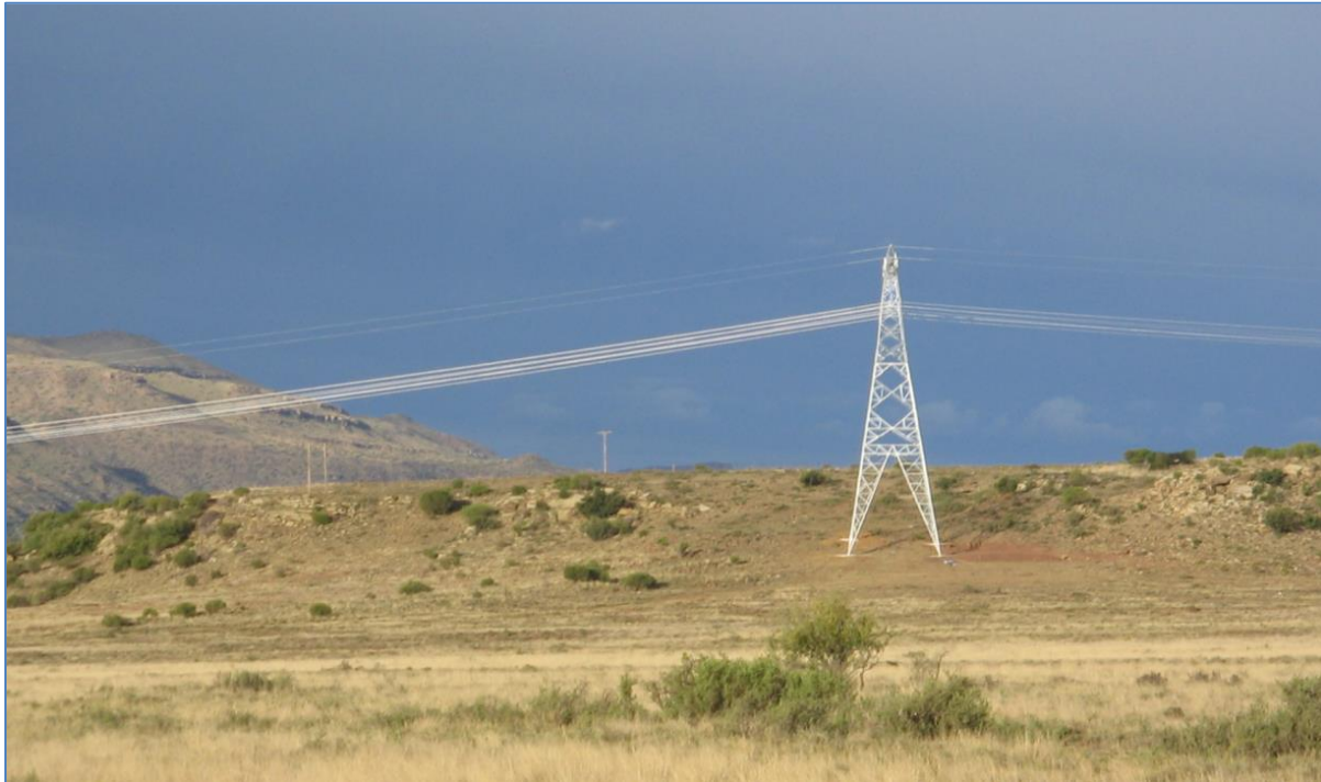
Figure 16. A 400 kV line, with all conductor wires in the same horizontal plane. This picture also demonstrates the almost invisible thin earth wire (black arrow) in top (Photo: EWT-WEP) (Prinsen et al. 2012).
