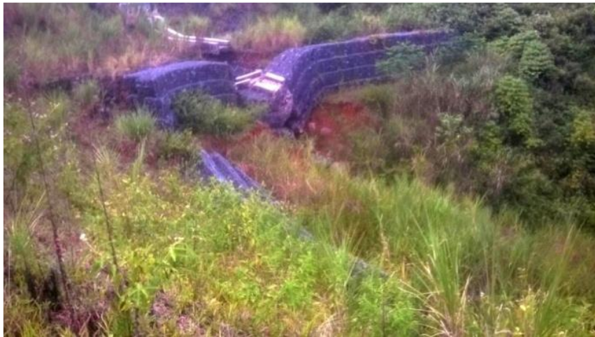
Figure 124 Landslides due to erosion in the area treated with gabion walls
