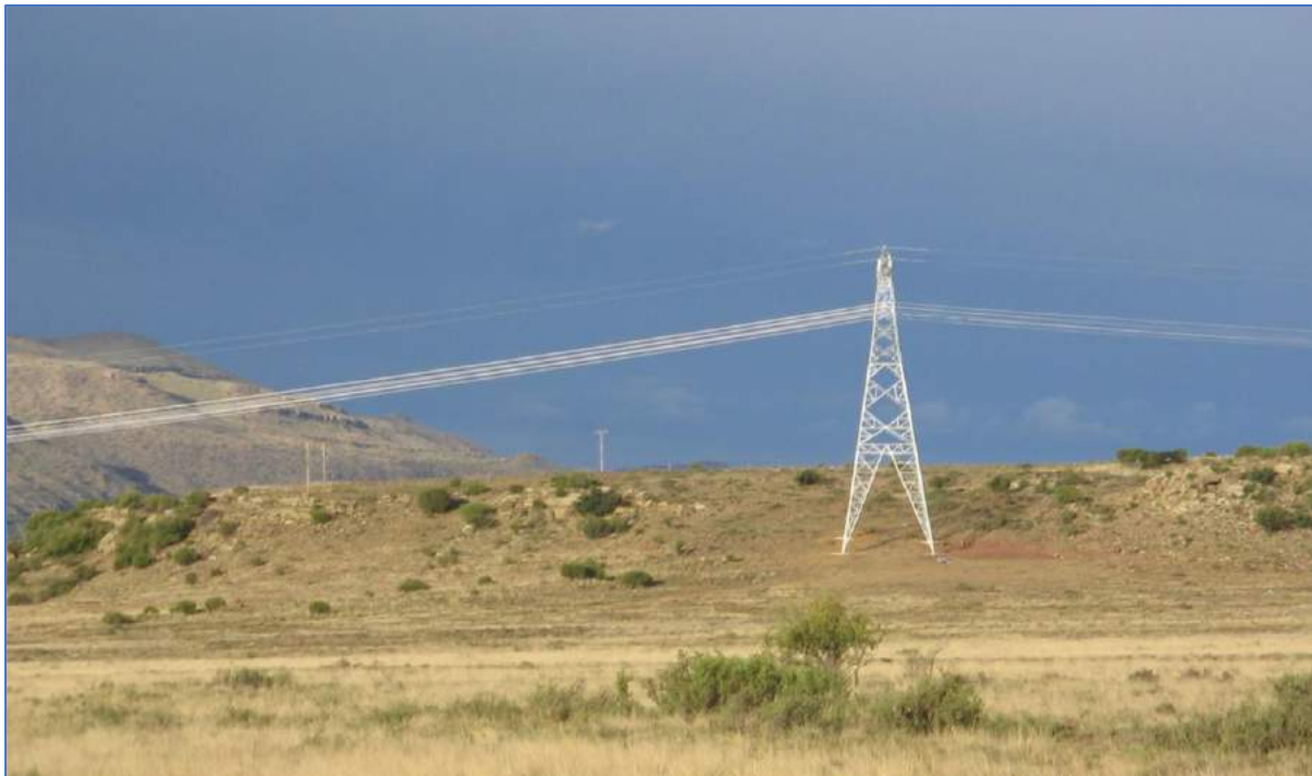
Figure 125. A 400 kV line, with all conductor wires in the same horizontal plane. This picture also demonstrates the almost invisible thin earth wire (black arrow) in top (Photo: EWT-WEP) (Prinsen et al. 2012).
